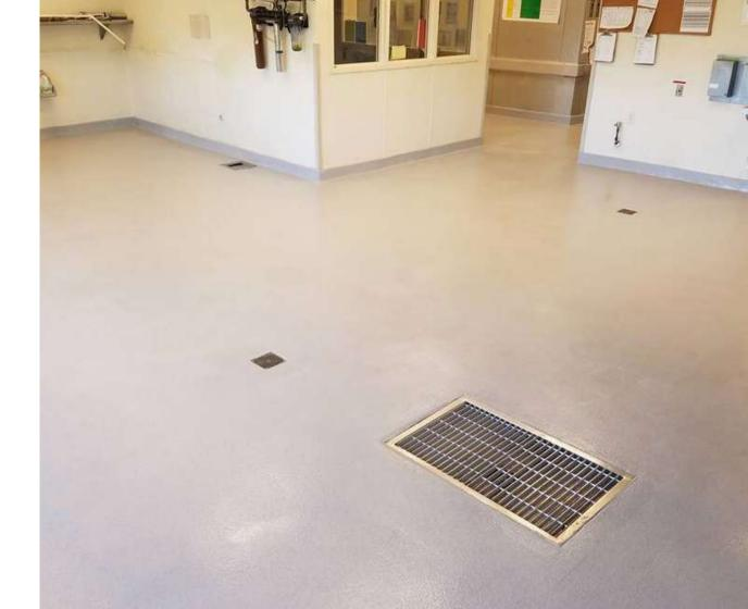
**Hermetic™ Quartz Floor** is a high build, double broadcast system using coloured quartz aggregate and sealed with a protective top coat.
