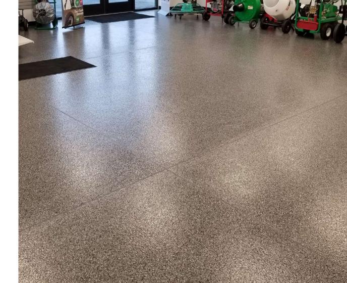
**Hermetic™ Flake Floor** is a durable, seamless, chemical resistant floor providing adjustable levels of slight texture and colour to match any design theme or surroundings.
