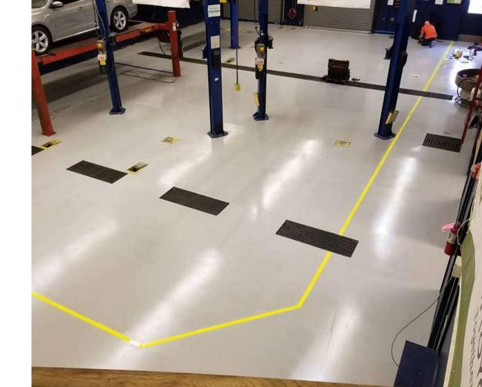
Hermetic<sup>™</sup> Neat Floor is a high build, self levelling clear or pigmented resinous flooring system engineered for industrial applications.
